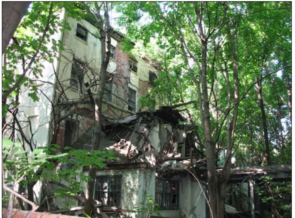
Rear (north) façade 2
