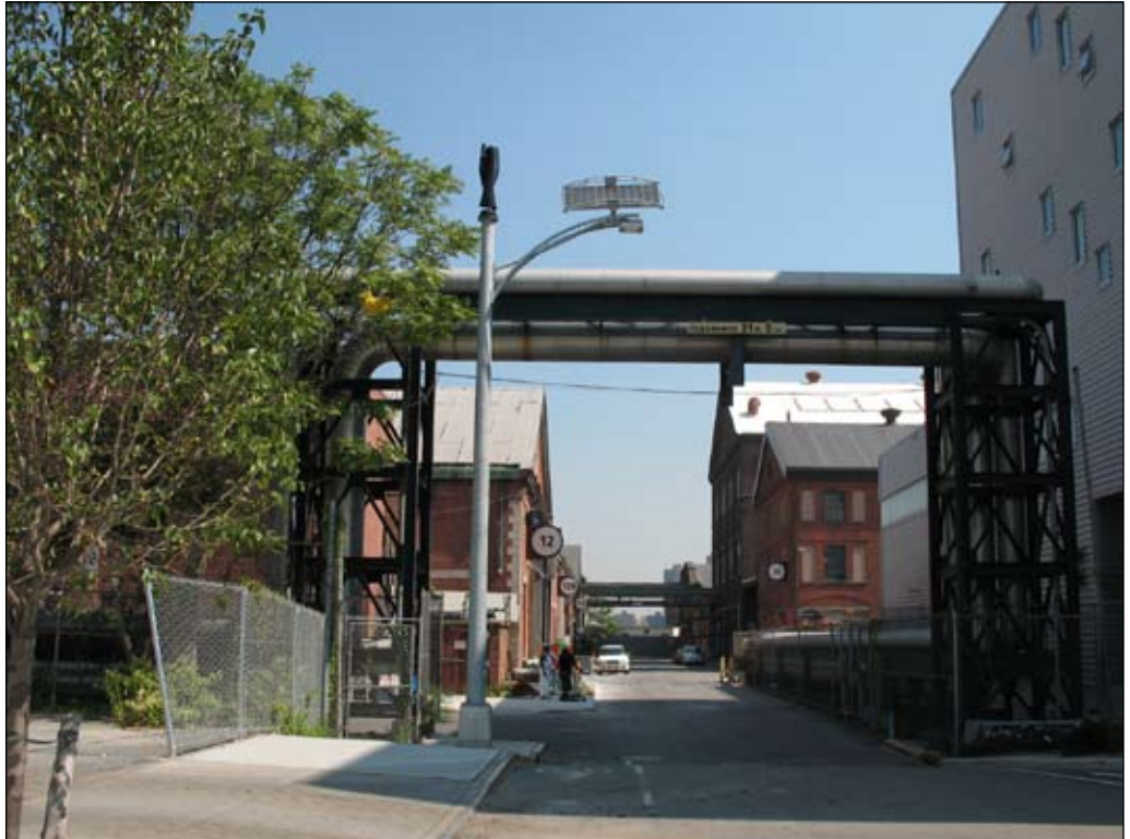
View northeast on Third Street from Chauncey Street. The recently constructed Building 25 is on the right 25
