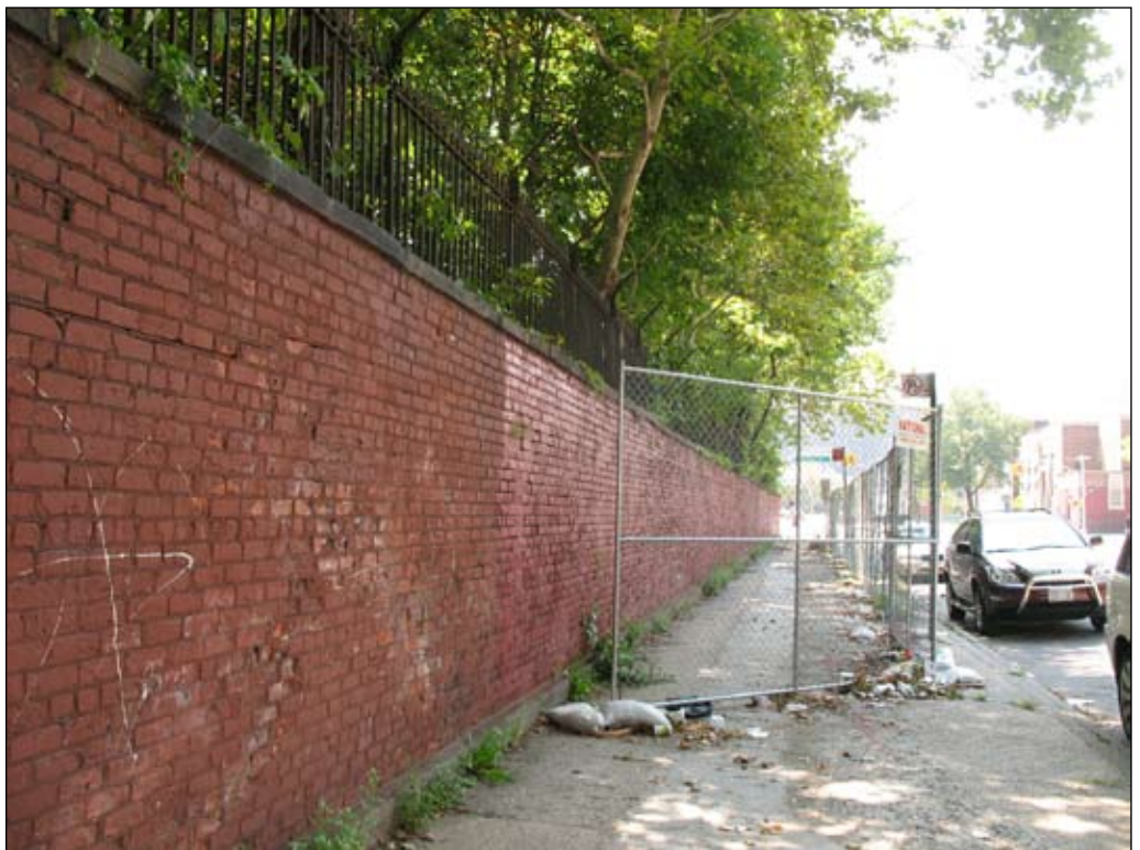
View south on Navy Street. The brick wall and iron fence that borders Admirals Row is on the left. The chain link fence on the sidewalk prohibits pedestrian access on the sidewalk by the Timber Shed, which has been determined to be structurally unsound 20
