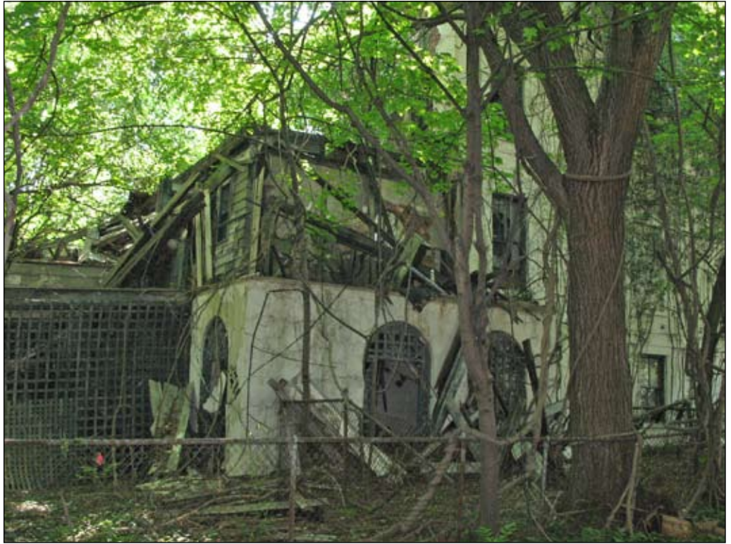
West facade of Building E 7
