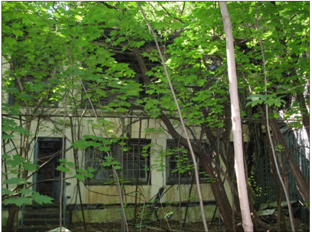
Rear (north) façade of Building G 8
