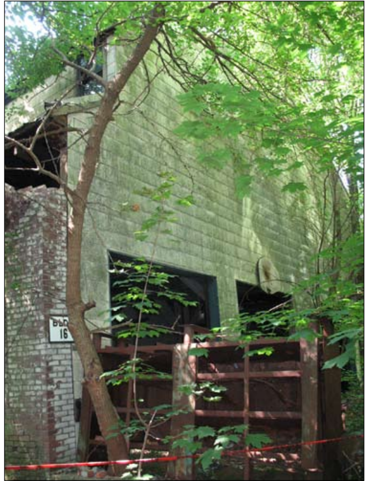
South (Park Street) façade 15
