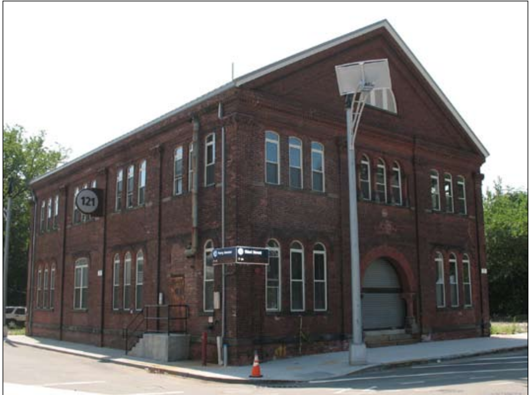
View southeast of Building 121. The Admirals Row site is located behind the building to the south 23
