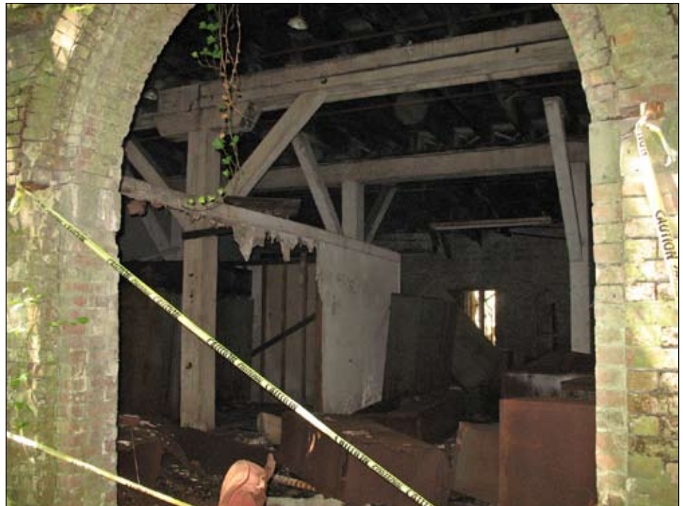
Timber Shed interior 16
