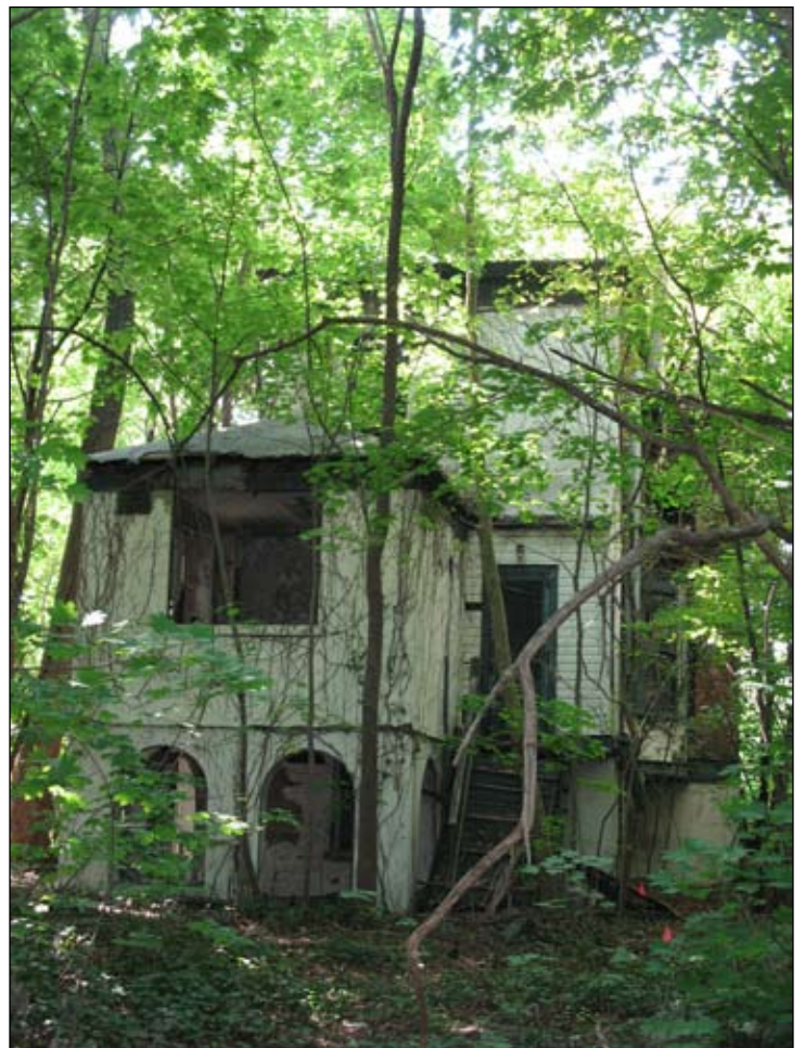
Rear (north) façade 12
