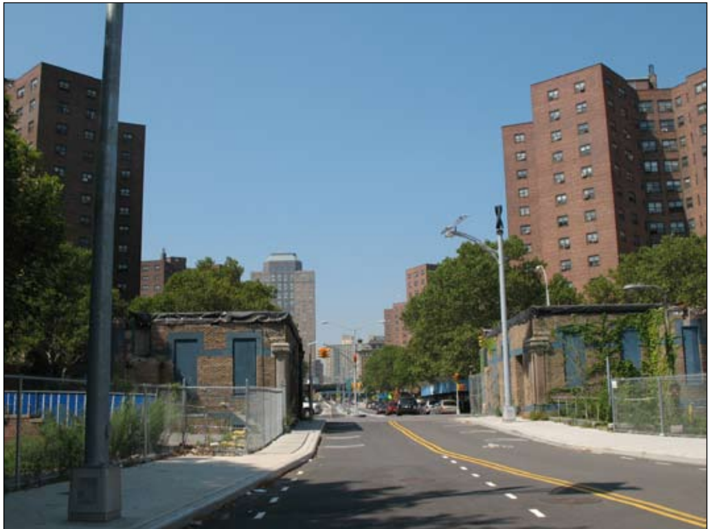
View west to Sands Street Gatehouse structures 26
